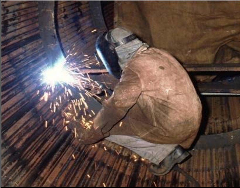
Figure Cutting and Welding Area
